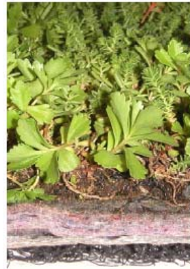
System Profile of the Xero Flor Extensive Green Roof Mats.
