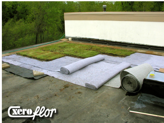
System Profile of the Xero Flor Extensive Green Roof Mats.
